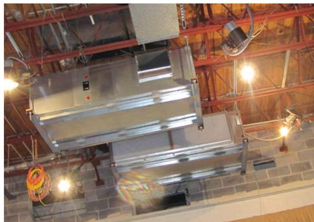
*Bosch FHP LV Series 8 and 10 ton commercial heat pumps installed in the ceiling of the auditorium. connect into existing ductwork system to provide year-round comfort*
