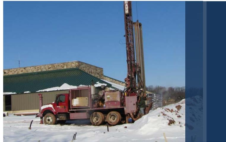
Twenty wells each 300 ft deep provide a closed-loop geothermal field routed to the mechanical room.
