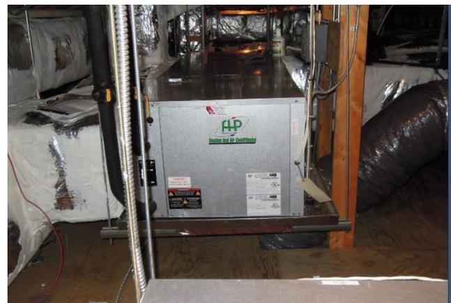
*Four 6 ton Bosch FHP horizontal geothermal heat pumps serve the 9,000 sq ft Kentlands Community Center to provide abundant heating and cooling*
